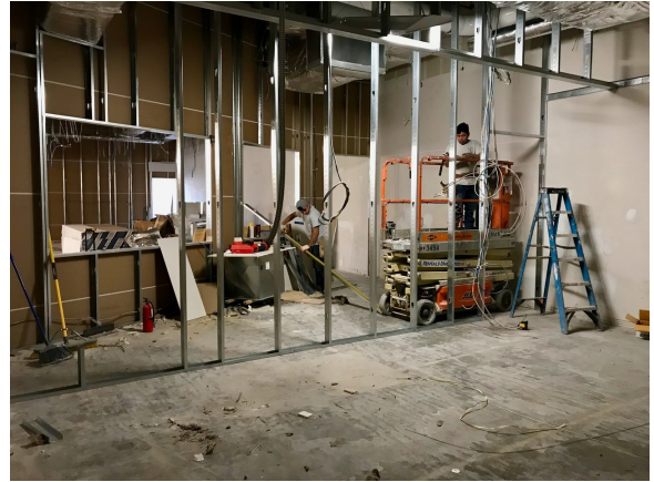
Workers install the wall between the cry room and the library.
